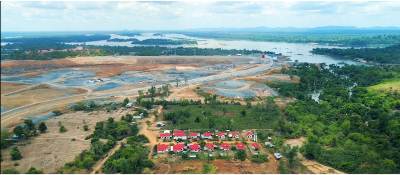
Don Sahong embankment structure image below:
