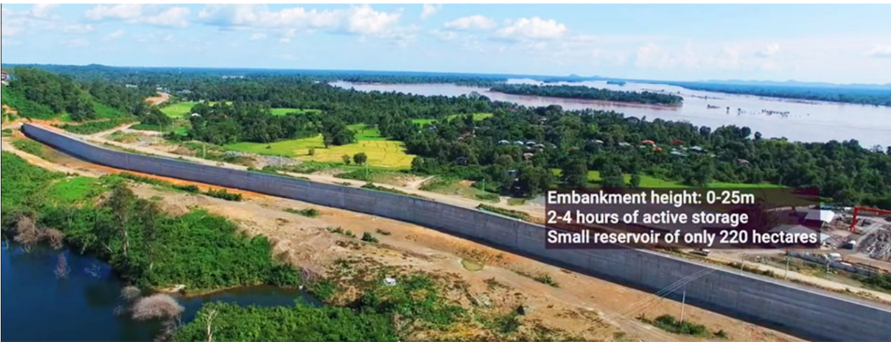
Don Sahong head pond channel dredging and embankment shown below:
